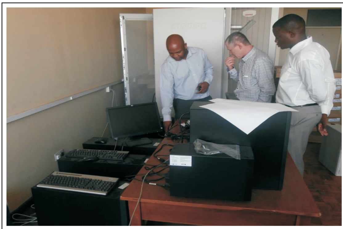
Figure 6. National server room hosting the new DHIS 2 system on one of the machines.
